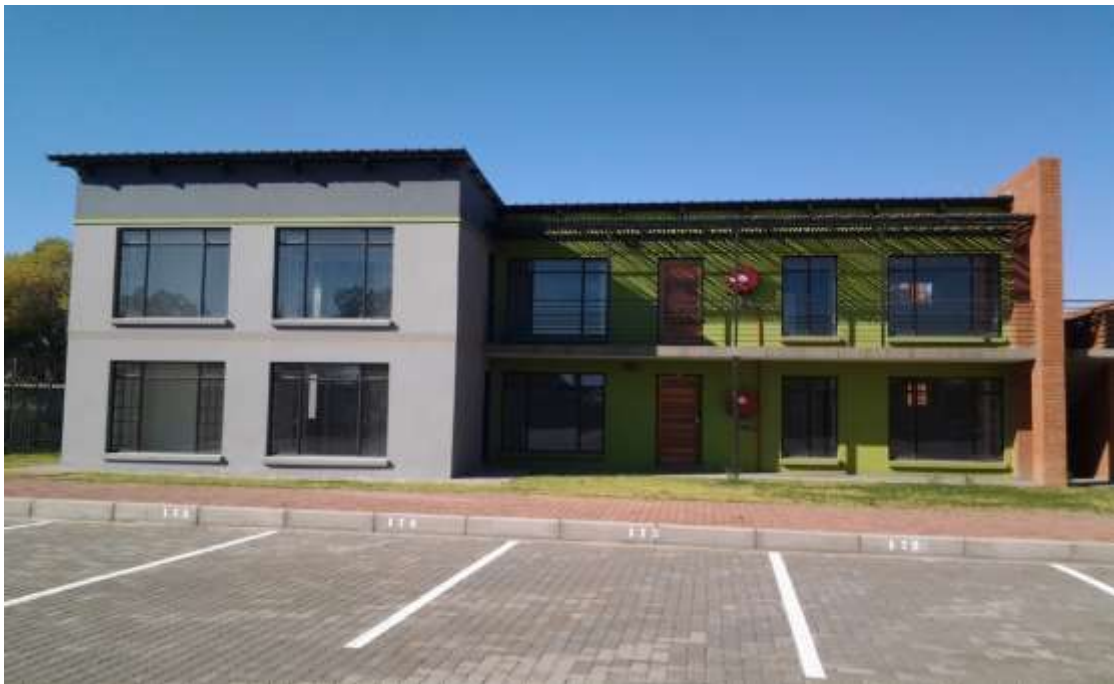
ZAMDELA CRU UNITS
