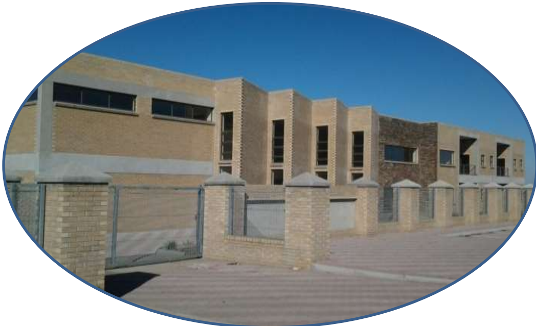
NEW MUNICIPAL BUILDING
